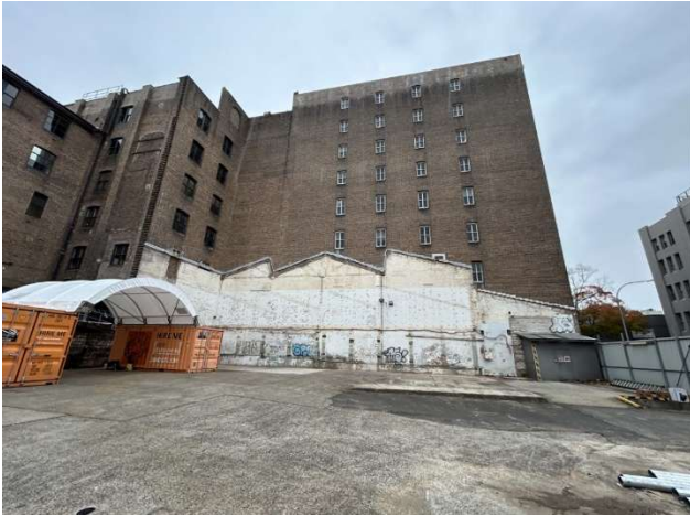
Figure 11 - View west showing the shadow profile of former buildings on neighbouring 1-3 Smail Street.
