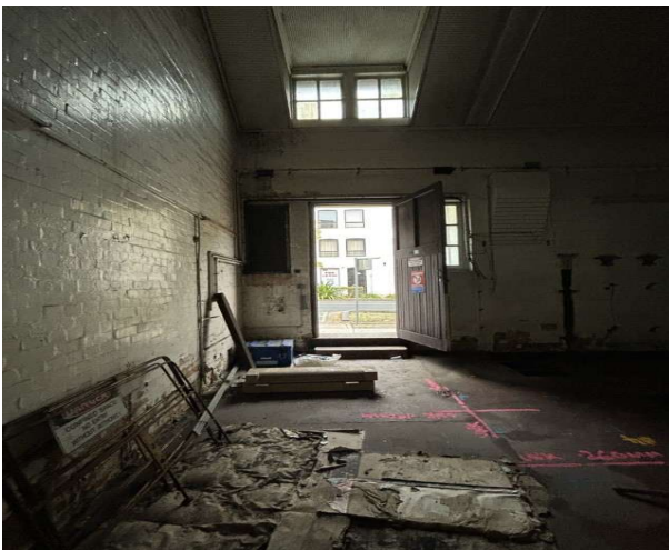
Figure 7 - View of dormer windows and entrance to the electricity Substation.
