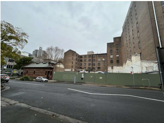
Figure 15 - View southeast toward the subject site. 55 Mountain Street is to the rear. And 1-3 Smail Street is at right
